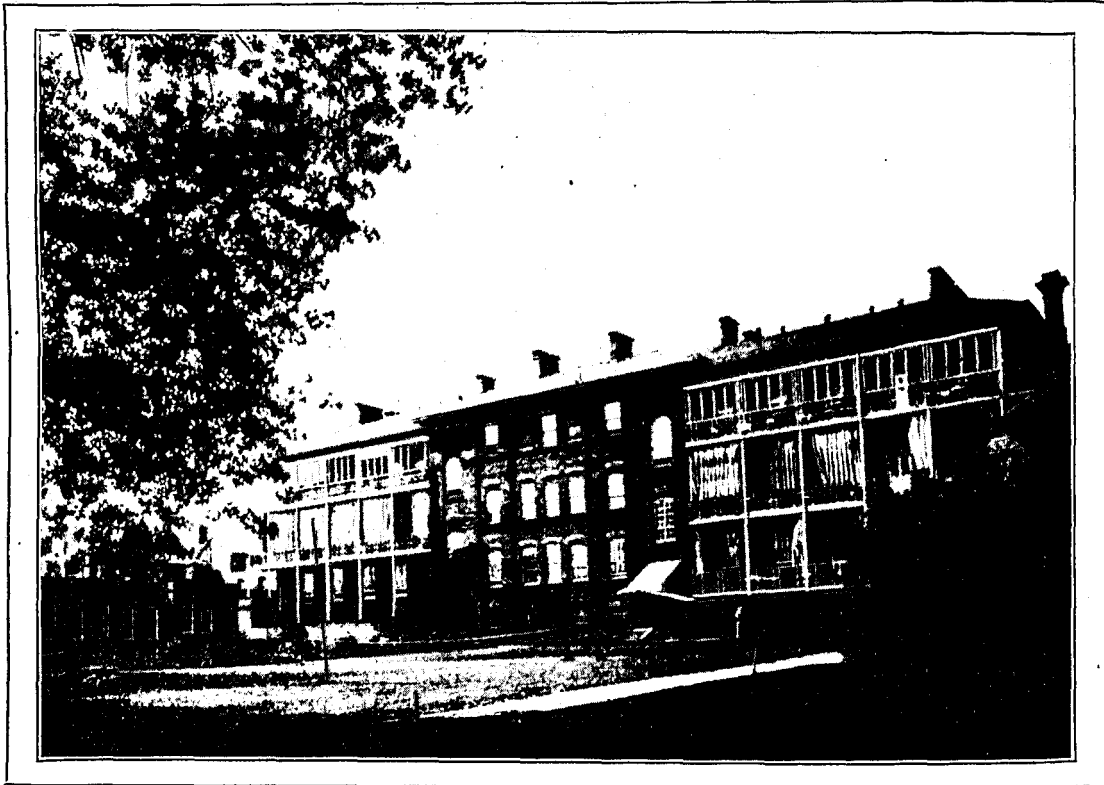
THE COUNTY HOSPITAL, YORK, SOUTH FRONT SHOWING BALCONIES.
